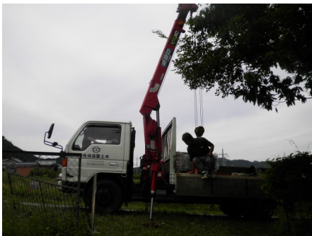
Hanairo Construction company in Kasai delivering stones and sand.
